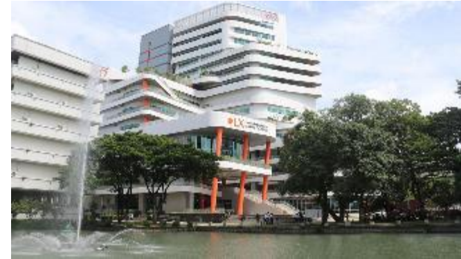
Learning Exchange Building King Mongkut's University of Technology Thonburi
