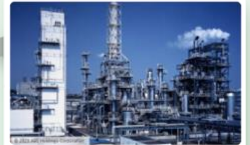
JGC Holdings Corporation IGCC Plant outside Indonesia
