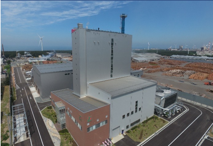
United Renewable Energy BTG 20.5MW
