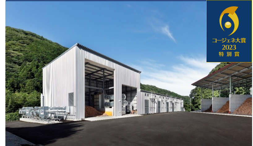
Tsuwano Forest Energy, CHP 0.5MW
