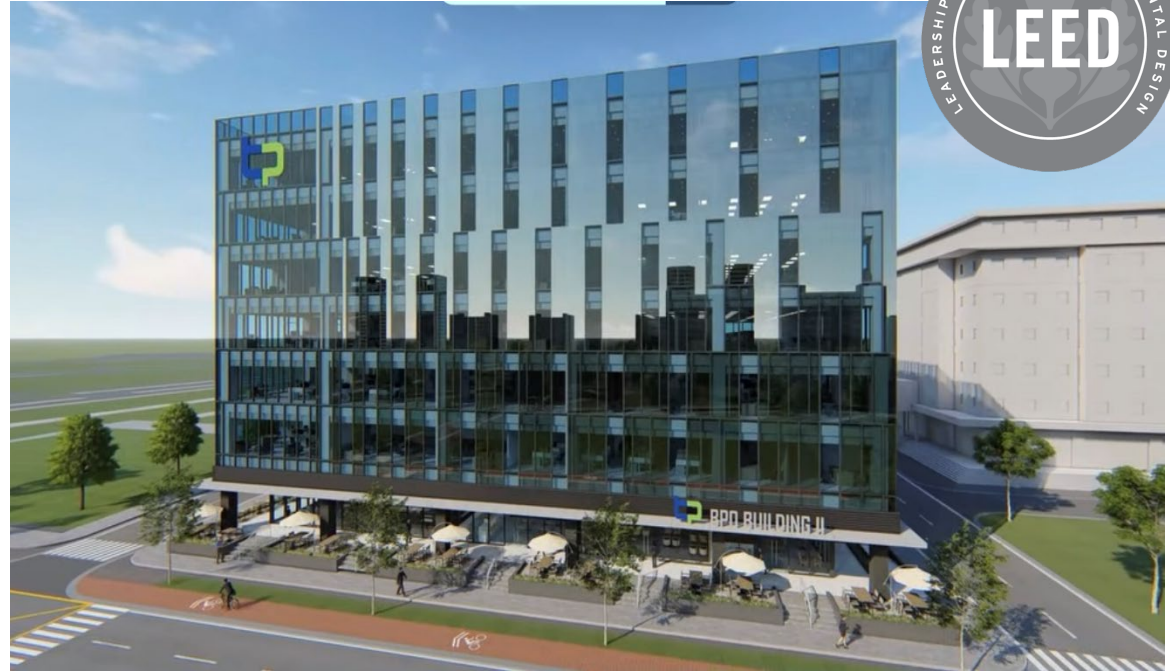
BPO Building Modification for LEED Certification (pipeline project)
