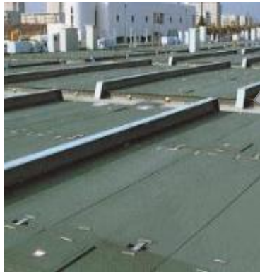
Treatment tank covers of sewerage (tie-up with Tokyo metropolitan government)
